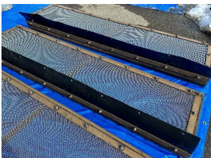
▲金網・防塵ゴムの更新
